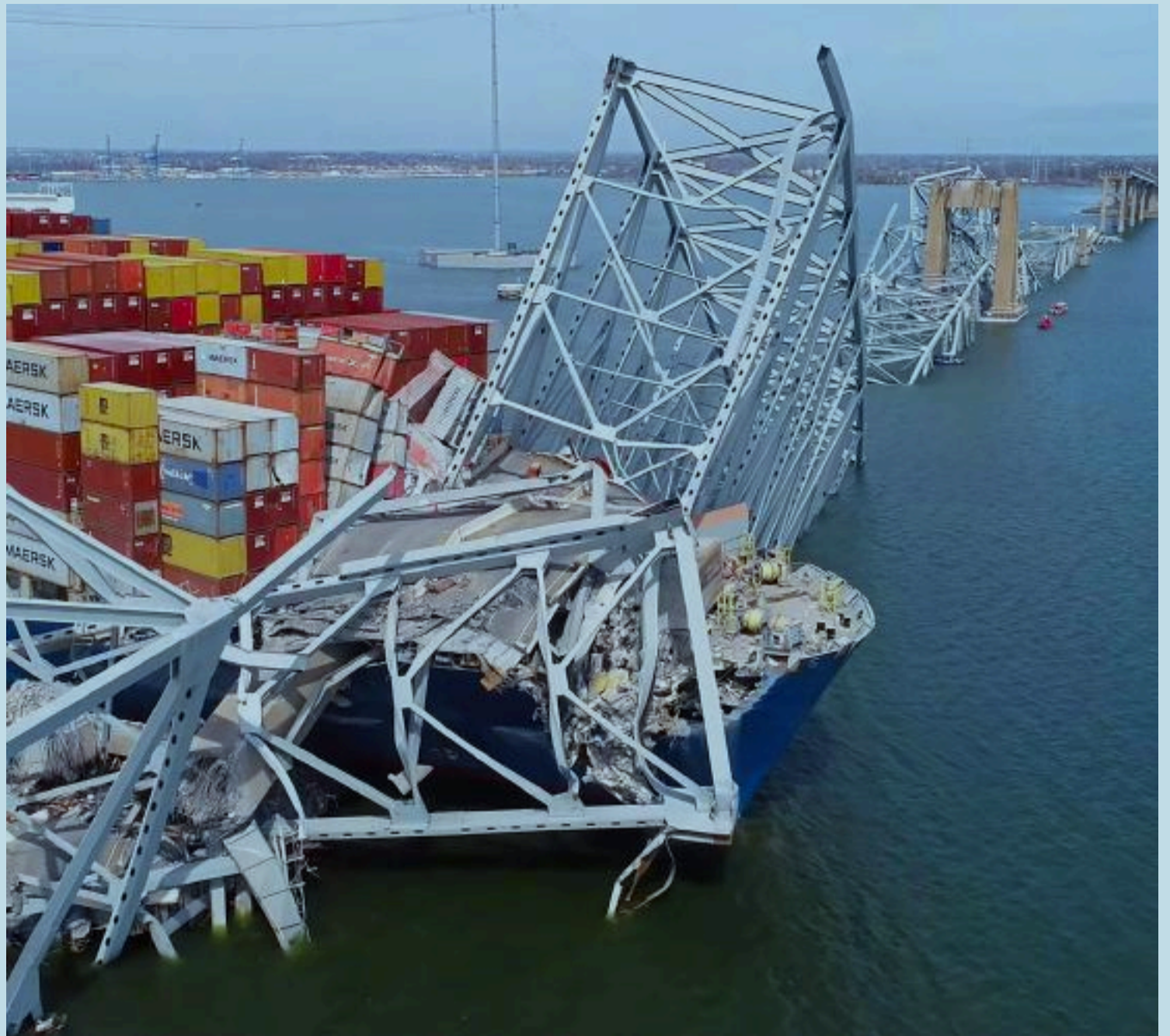
BREAKDOWN: The main spans of the Francis Scott Key Bridge in Baltimore tumbled after the 9,962-teu Dali (built 2015) struck one of its support pillars Photo: National Transportation Safety Board
