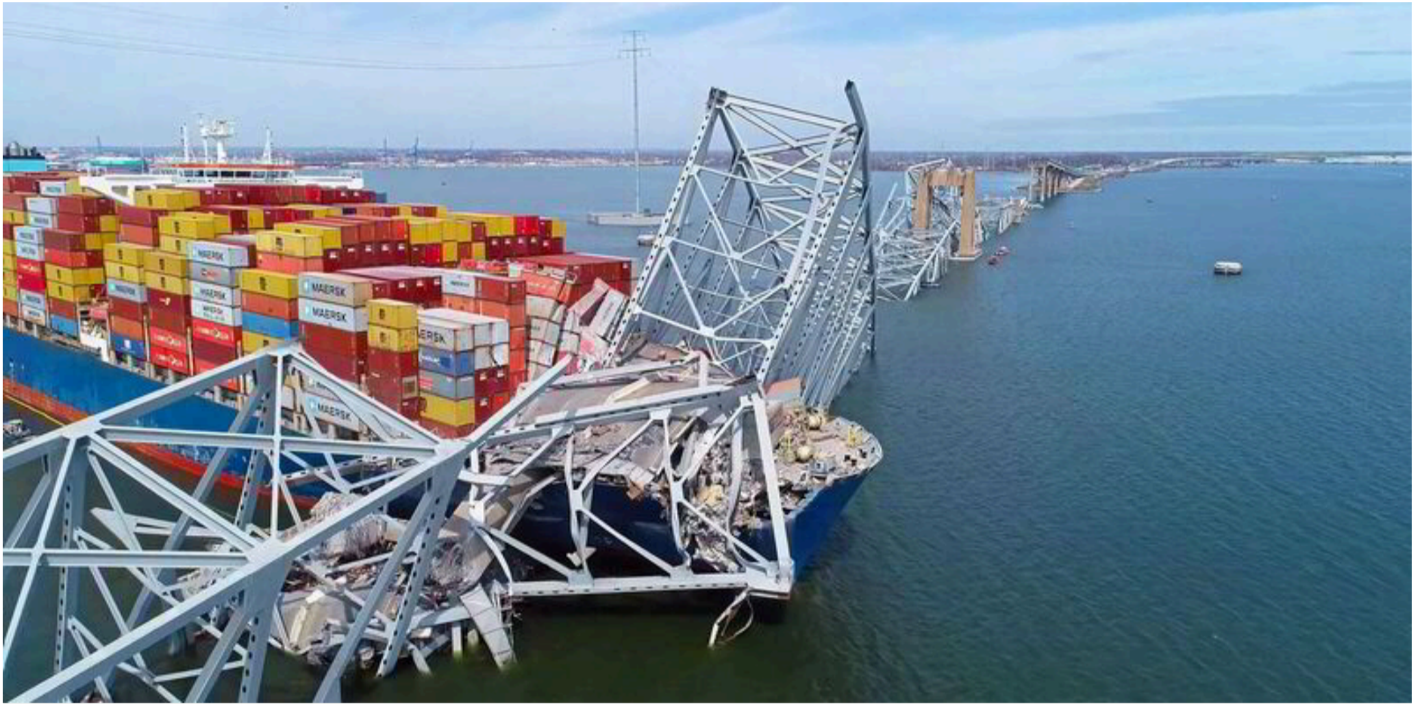
The main spans of the Francis Scott Key Bridge in Baltimore collapsed after the 9,962-teu Dali (built 2015) struck one of its support pillars. Photo: National Transportation Safety Board
