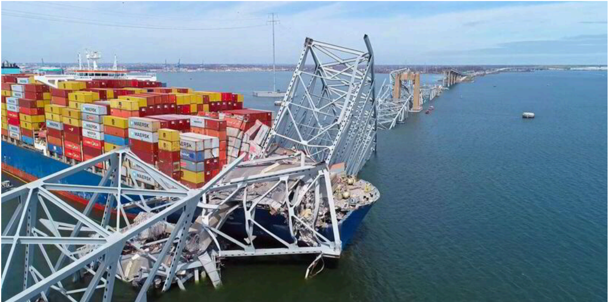
The Francis Scott Key Bridge in Baltimore collapsed in March after it was hit by the Dali. Photo: National Transportation Safety Board
